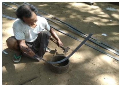
Fig.3.1.1 (a) Cutting and bending iron rods
