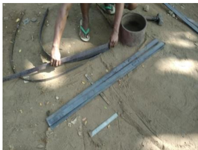
Fig.3.1.1 (a) Cutting and bending iron rods
